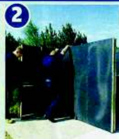
2 Deano Eley and Bradley Glover start with the walls.
