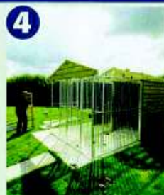
4 And now for the roof rafters and trusses...
