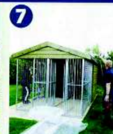
7 ...before hosing down the roof to check the guttering.
