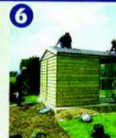
6 Dean (snr) applies a marine sealer to the woodwork...
